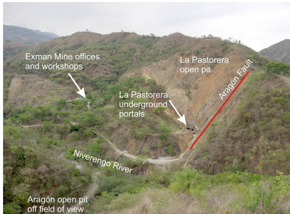
Figure 5.2 View of the La Pastorera open pit and the mine offices (Source: Snowden site visit 2010)
